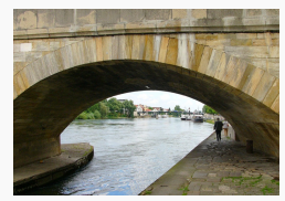
Stone Bridge detail
