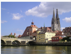
Bridge tower and Salt shed
