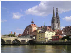
Bridge tower and Salt shed
