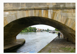
Stone Bridge detail
